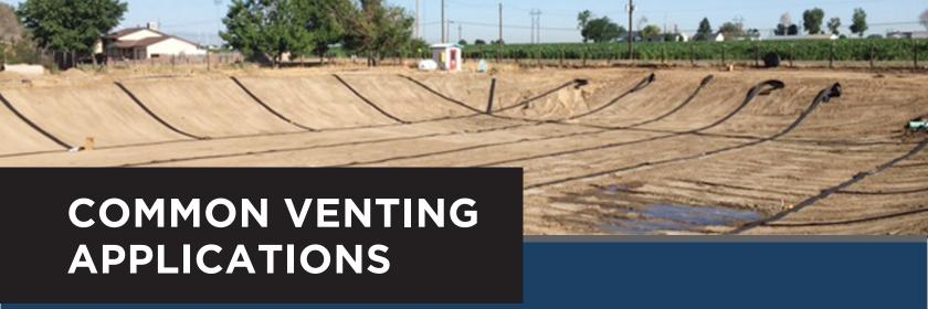
Utilizing the Hydravent Ventilation System, the Hydraway 2000 can be installed beneath pond and lagoon liners to act as a vent to protect from damage caused by methane gas and water accumulation.
